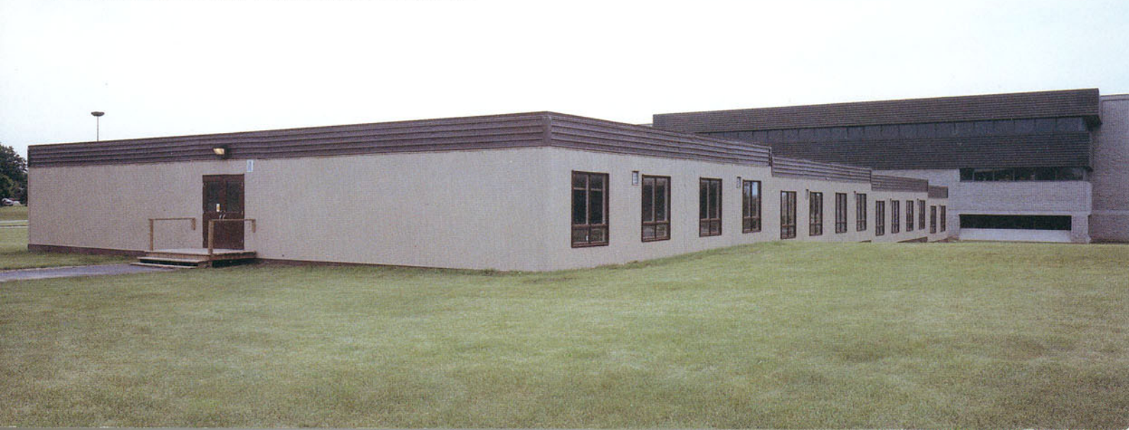
Centennial College, Scarborough – 15 unit relocatable classroom addition
