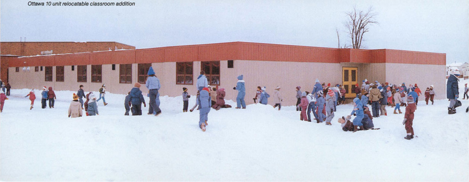
Ottawa 10 unit relocatable classroom addition
