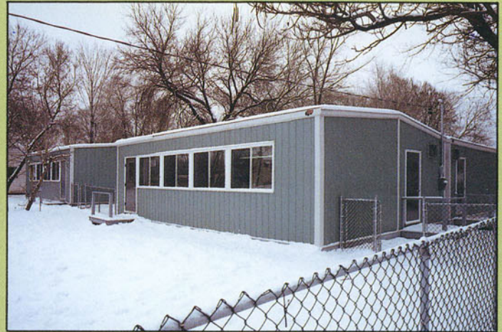
Typical four unit complex – Froebel Kindergarten, Mississauga
