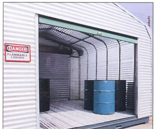
Hazardous materials storage building with two roll-up doors and open grate steel floor with reservoir for accidental spillage.
