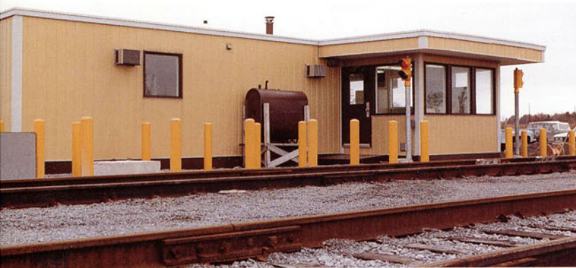
building for controlling rail and vehicular traffic.
