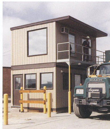
Sentinel two-storey check point for manifests and loads.
