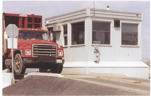
Sentinel security and weigh scale building.
