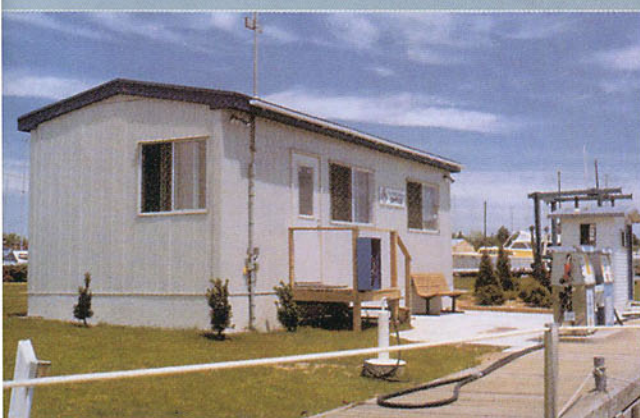
CPS Marina management office – Port Whitty
