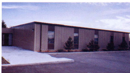
Halton Separate School Board office expansion.
